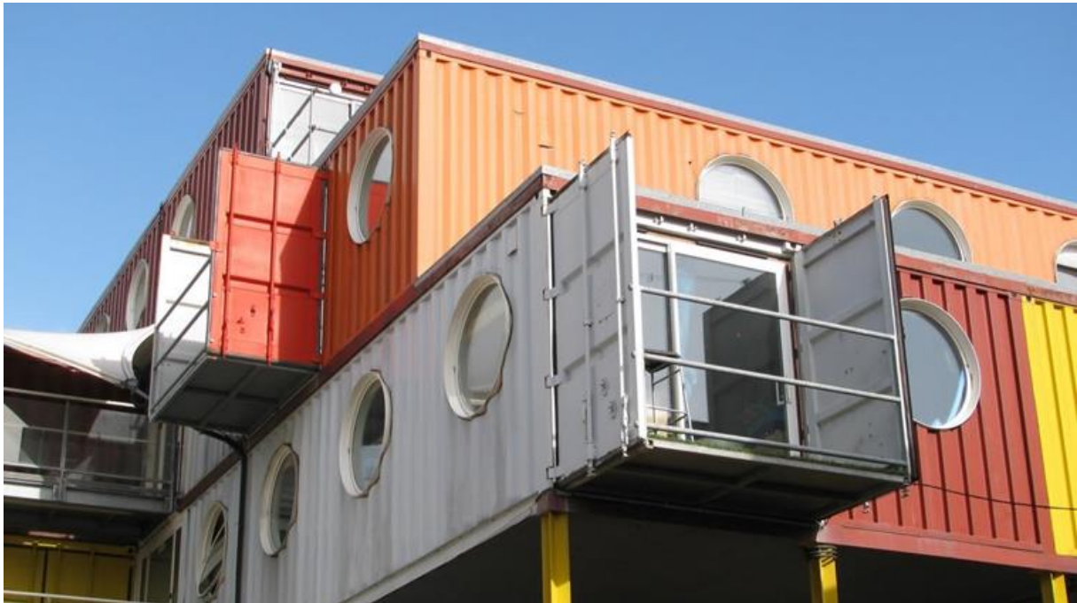
Figure 6: Work spaces from transformed 40-foot shipping containers.
