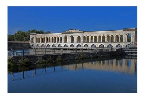
The dam allows to the Ticino river to be redirected towards two important canals: the **Industrial canal**, used for the production of electricity, and the **Villoresi canal**, used for irrigation purposes.
